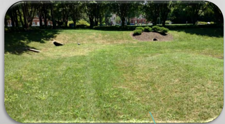
Inlets at end of berm
